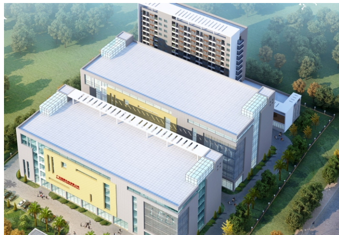
万润科技松山湖生产研发基地A区 建筑面积: 46106 平方米 LED照明研发与生产基地 A area of Songshan lake production research and development base of Mason Technologies Co., Ltd Construction area: 46106 Square meters LED lighting production research and development base
